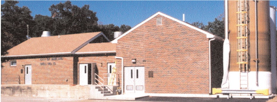
Well # 13 - 1400 GPM Radium Removal Facility
