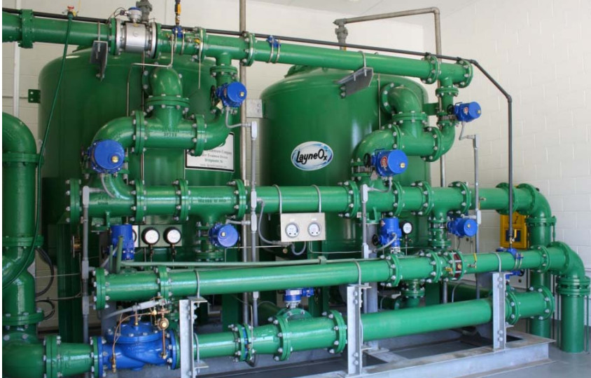
LayneOx operates as both a classical filter working with an oxidant and as a catalytic media.
