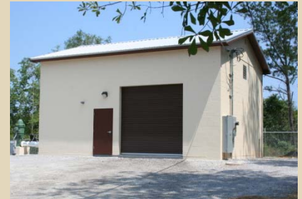
The LayneOx design is less expensive to construct as the improved performance provides financial benefits in the form of a smaller building.
