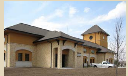
Exterior of the Hutchinson Water Treatment Center. The clock tower conceals a degasifier.
