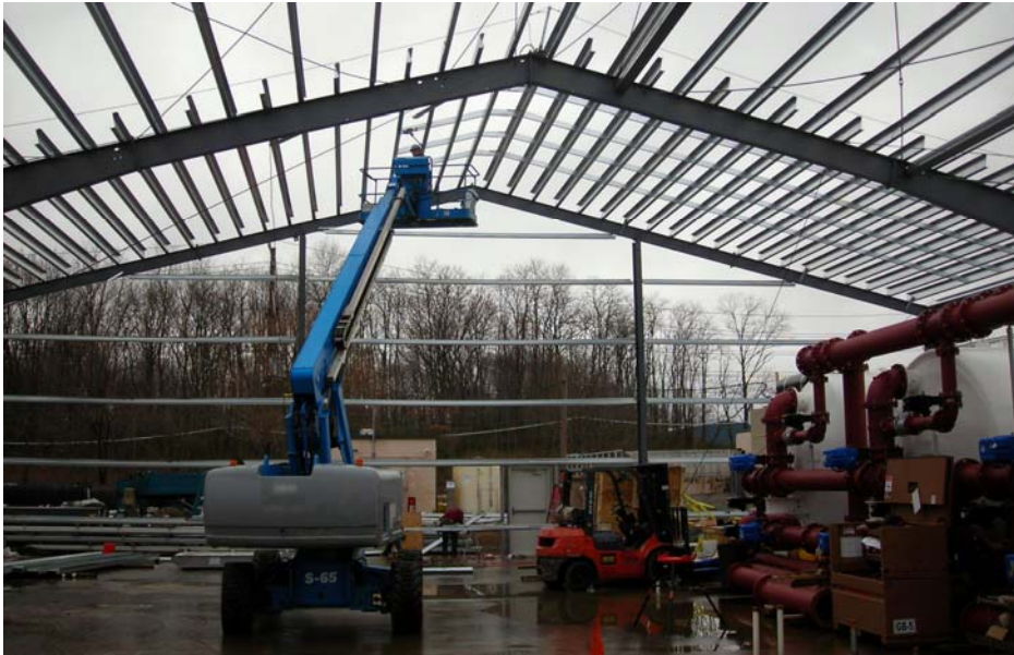
New Water Treatment Plant mid-construction. Note multi-media filters on far right.
