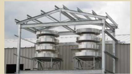
Cascade Aerators oxygenate raw water.
