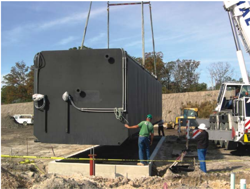
Layne crew installs a Fluidyne ISAM at this Lewes, Delaware subdivision.
