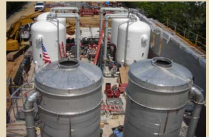
Overhead view during construction shows air strippers in foreground.
