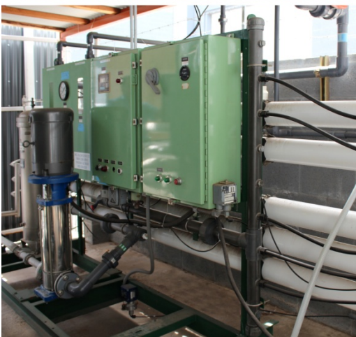
DI and RO systems maintained by Layne Christensen provide high purity water for Entrepix operations.
