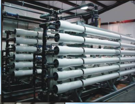
Layne can design, build and maintain specialized treatment equipment such as this membrane and pressure filter installation in Phillipsburg, Kansas.
